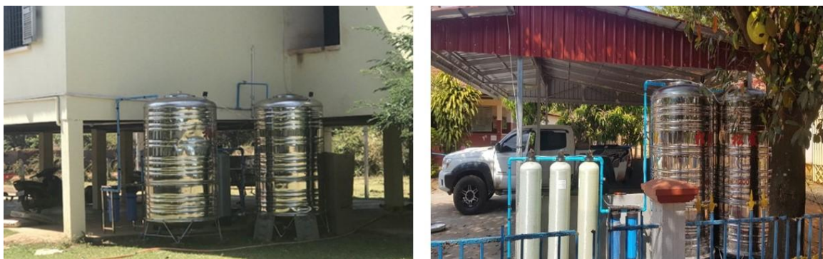
Figure 43: The installation of water treatment equipment in health centers in Ratanakiri province. Source: (WHO, 2021)
