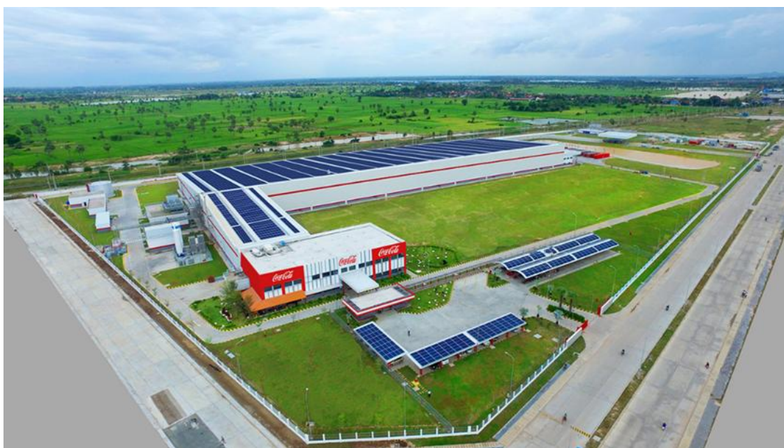
Figure 41: The installation solar rooftop for energy supply in the factory. Source: (B2B Cambodia News, 2017).
