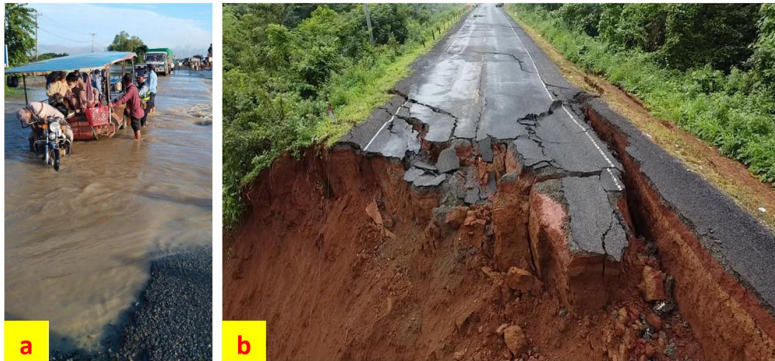
Figure 35: Road infrastructure damaged by floods: a) flood damaged National Road no. 5 and b) heavy rain damaged National Road 76 at Mondulkiri province. Source: (Cambodia News, 2023).
